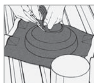
1. Adjust Dektite® to the pipe.
